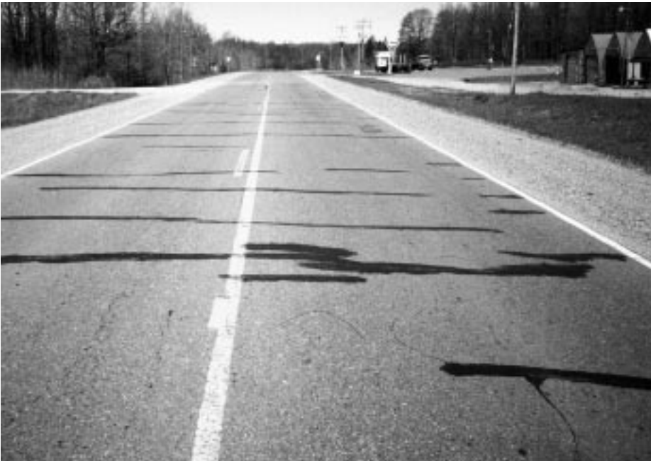
◀ Sealed cracks, a few feet apart.
